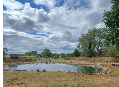
Large Pond Installation - Aug 23
