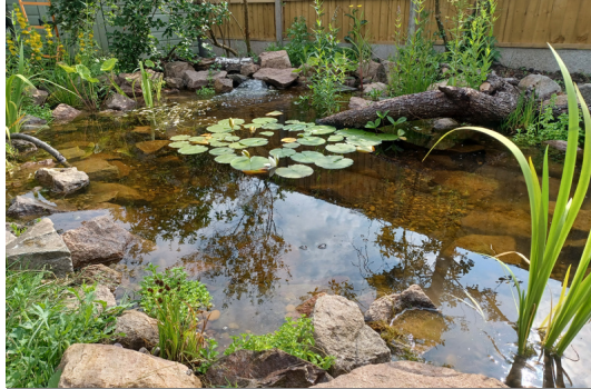
Eco Pond & Waterfall Installation - April 23
